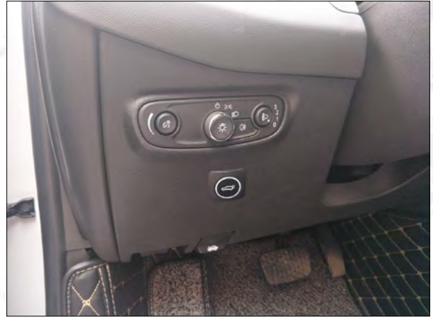
10. Under the main driving, remove the trim panel, punch and install our front switch button.
